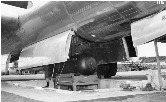
Loading 'Thin man' into Enola Gay before Hiroshima. The bomb is first lowered into the pit, the B-29 moved over it and the bomb raised by a large vertical hydraulic ram. See http://tinyurl.com/mrgtmau for many more photos.
